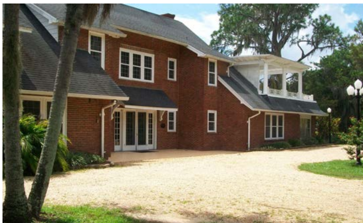
The Mackay House as it looks in 2020
